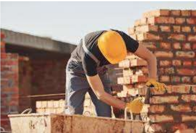
Brick Wall Work
