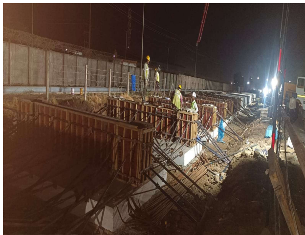
Pedestal Casting Work For Mechanical Structure
