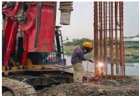
Reinforcement Work for pile Cage
