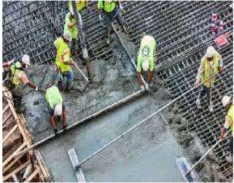
RCC Finishing Work
