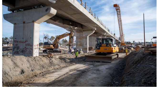
Bridge & Service Road Work
