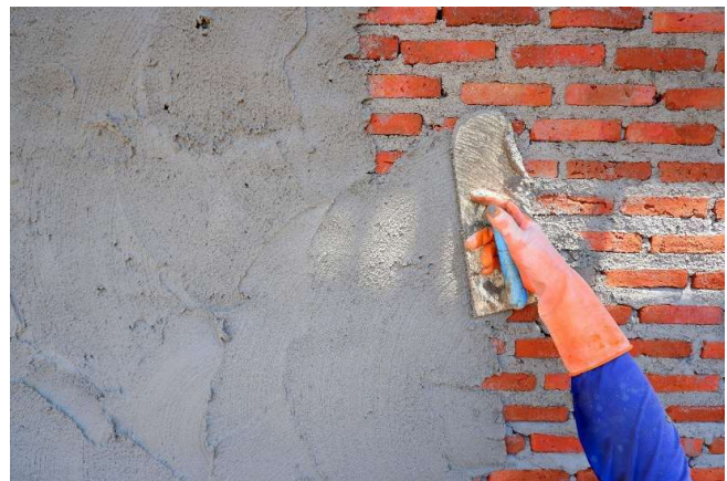
Plaster Work / Finishing
