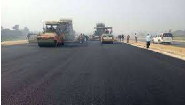
Bituminous Road Work
