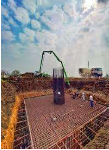
Pile-Cap Concreting work
